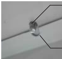
Threaded Stud on HOUSING
